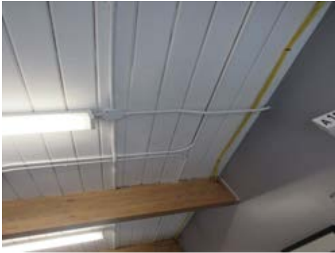
SURFACE MOUNT BANANA CABLE FOR ACCESS CONTROL.
