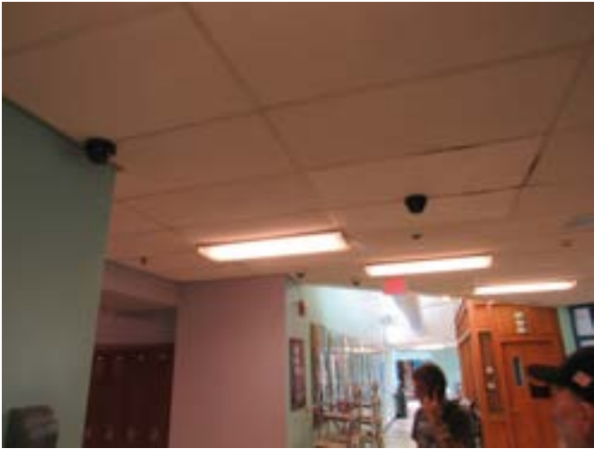
MULTIPLE CAMERAS AT A SINGLE APEX INTERNALLY
