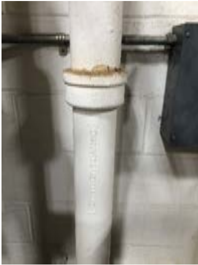
Hub & Spigot Cast Iron Vent Pipe
