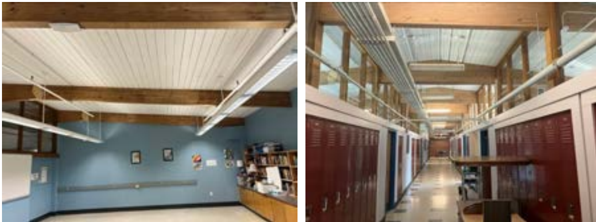
Typical Roof Framing of the Original Structure
