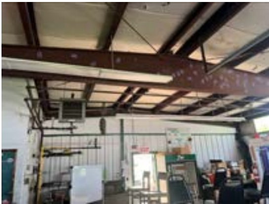
Typical Framing of the Horticulture Bldg. Roof and Greenhouse
