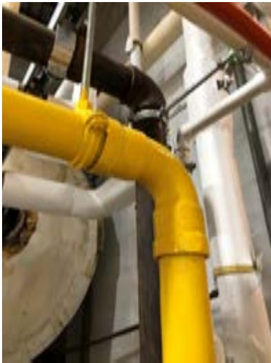
Pressed Gas Pipe Fitting
