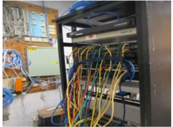
NO COHESIVE COLOR CODING TO PATCH CABLES FOR SYSTEMS.
