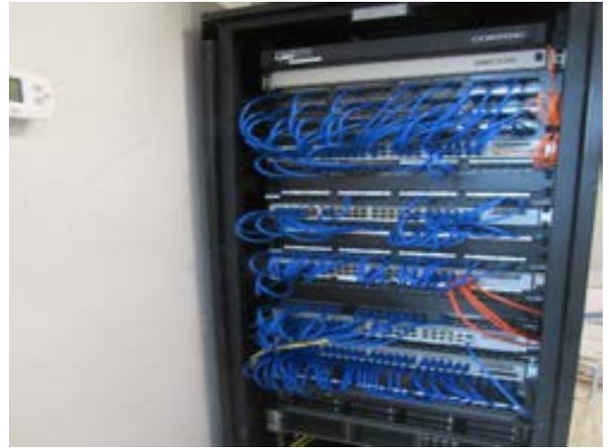
MORE CLEAN CABLE INSTALLATION
