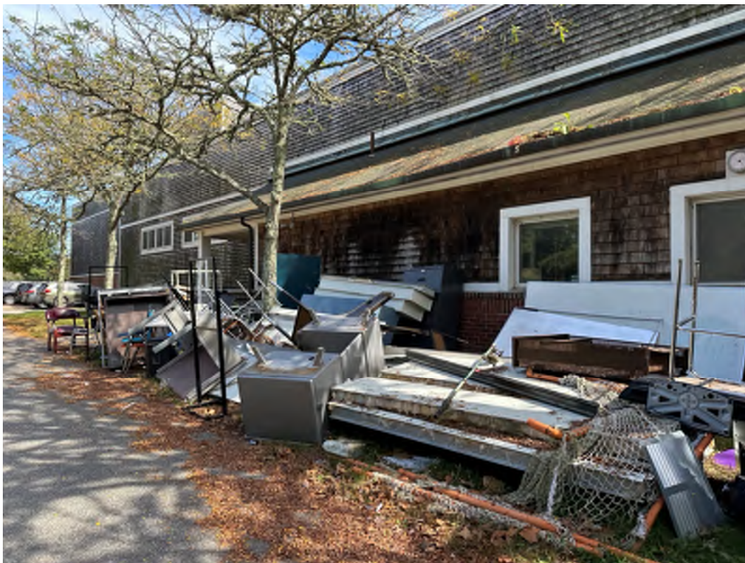
Photo 24: Scrap metal storage on western side of building.
