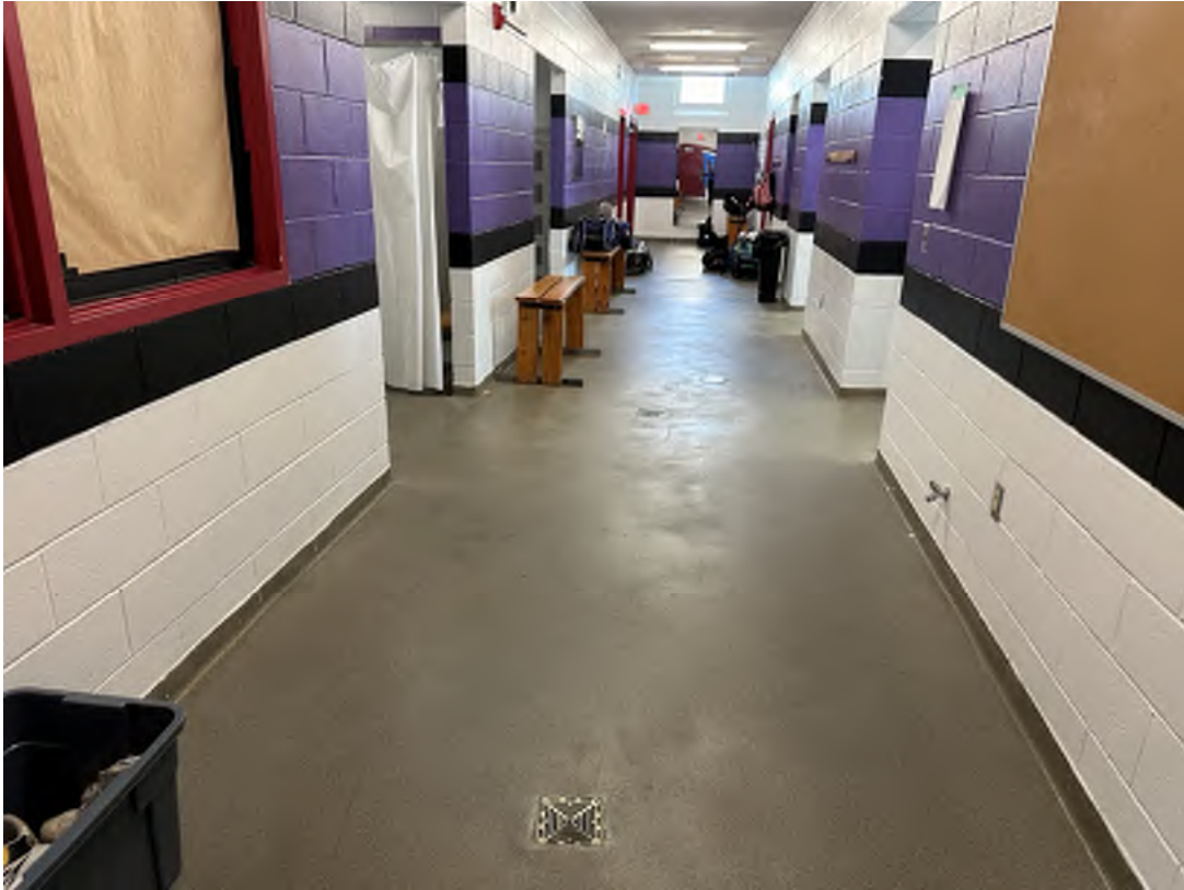
Photo 9: Floor drains observed in locker rooms.
