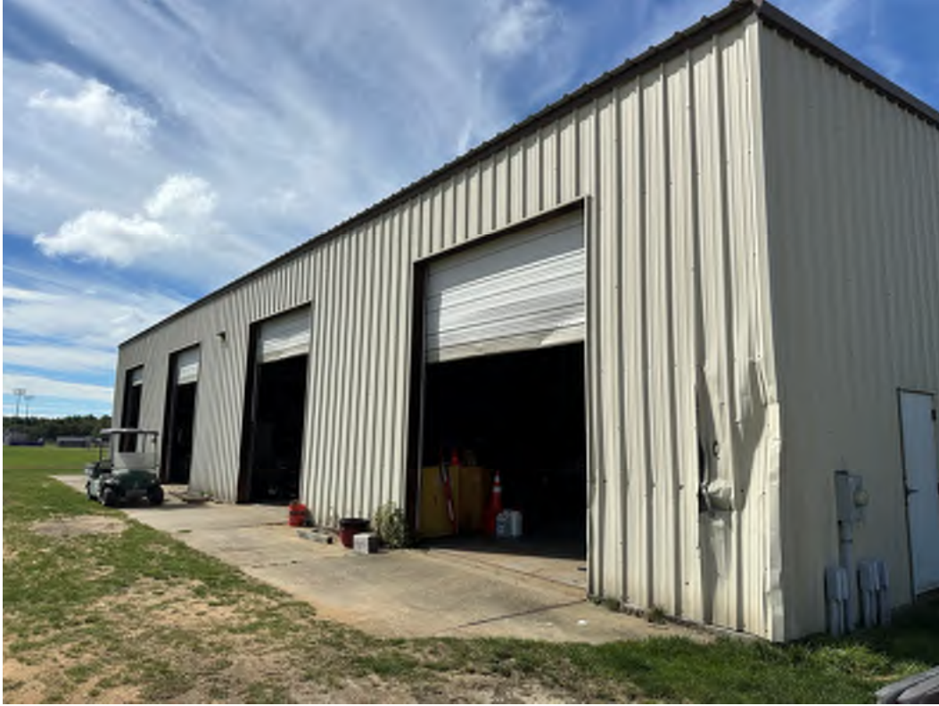
Photo 21: View looking south at maintenance garage.
