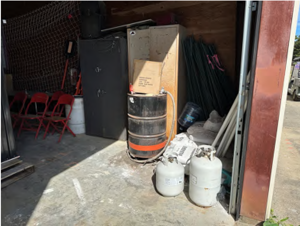
Photo 19: 55-gallon drum of methanol and liquid propane storage in maintenance garage.
