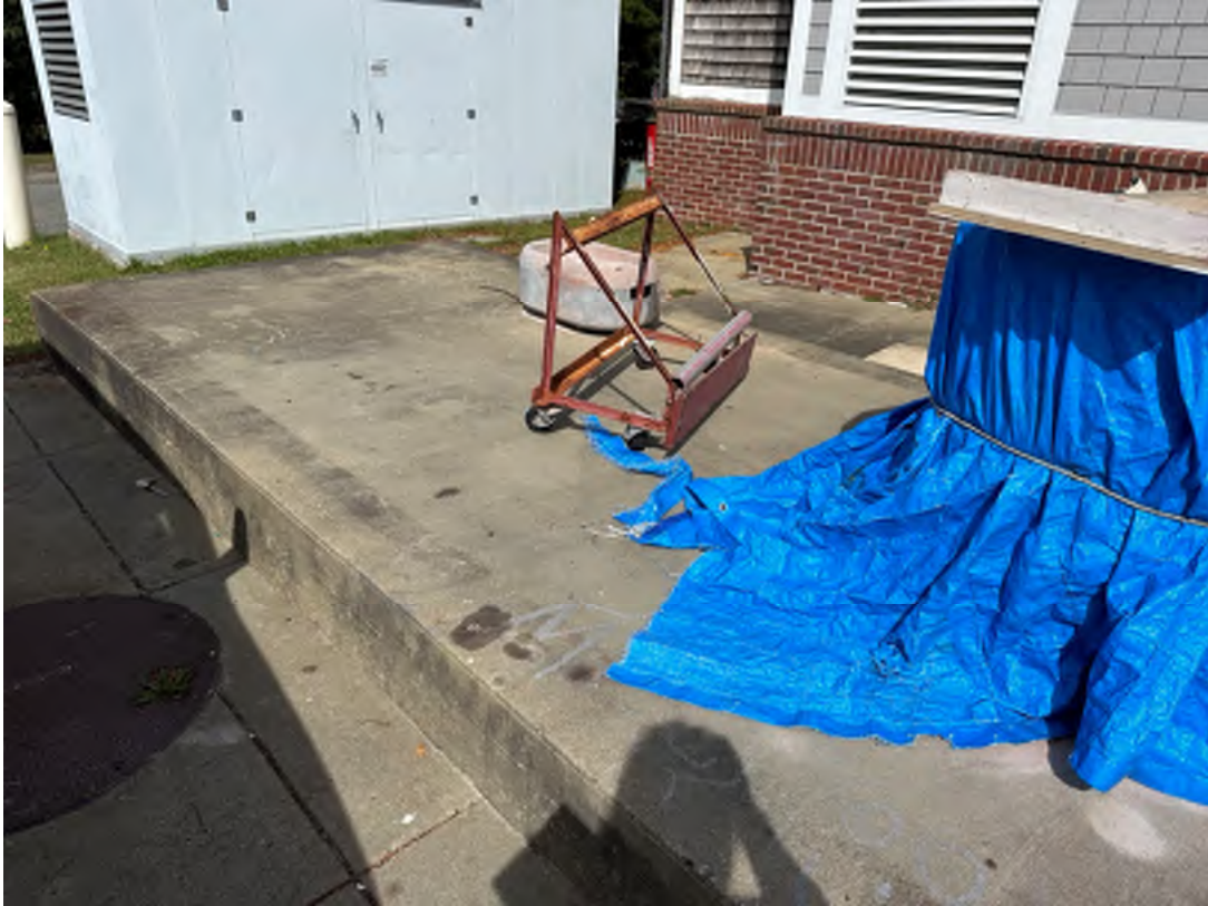
Photo 13: 10,000-gallon UST located adjacent to backup generator.
