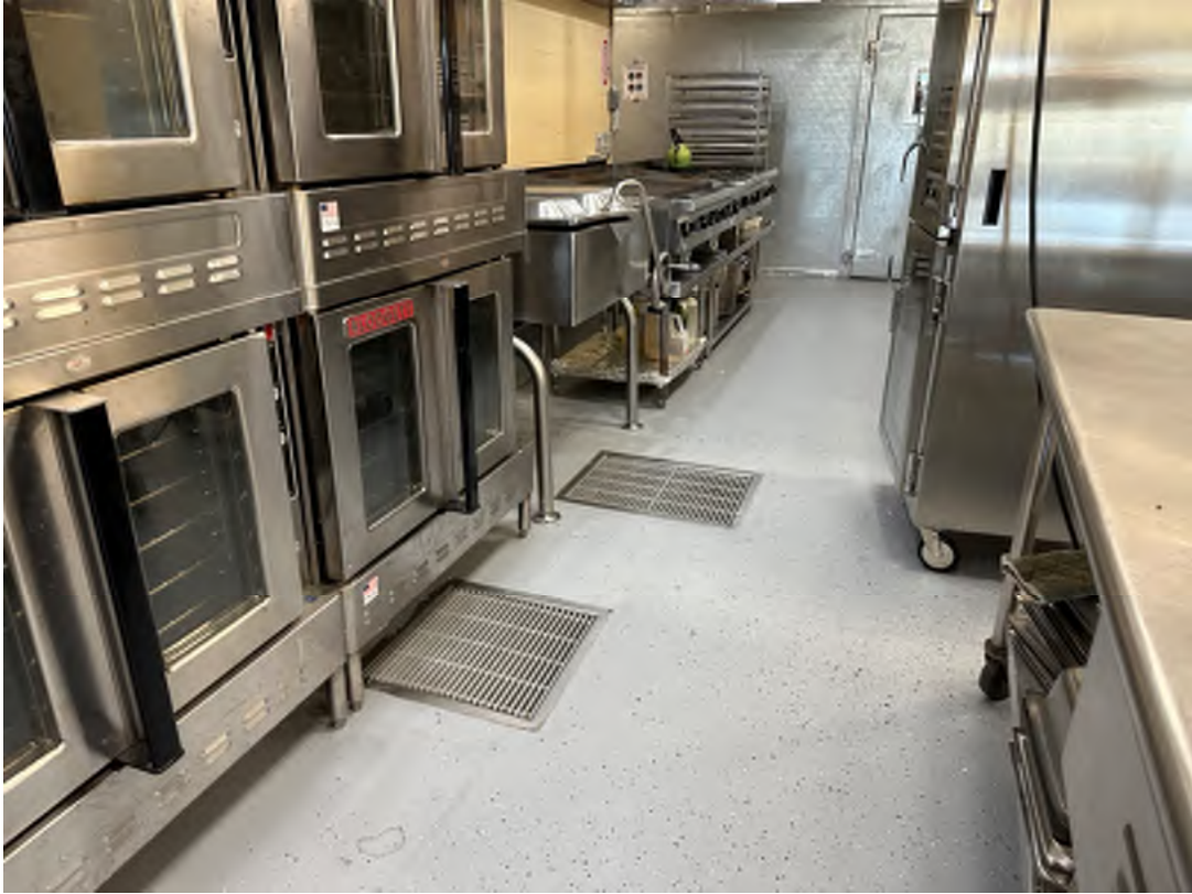
Photo 15: Floor drains observed in cafeteria kitchen.
