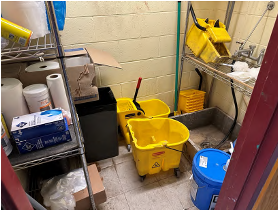
Photo 14: Maintenance closet with floor level sink.
